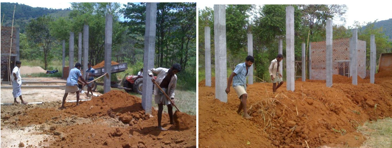
Gravel soil been unloaded and spread for the cattle shed floor
